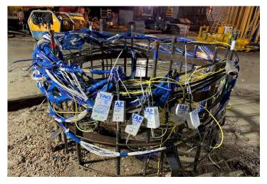
Thermal Integrity Profiling loggers
